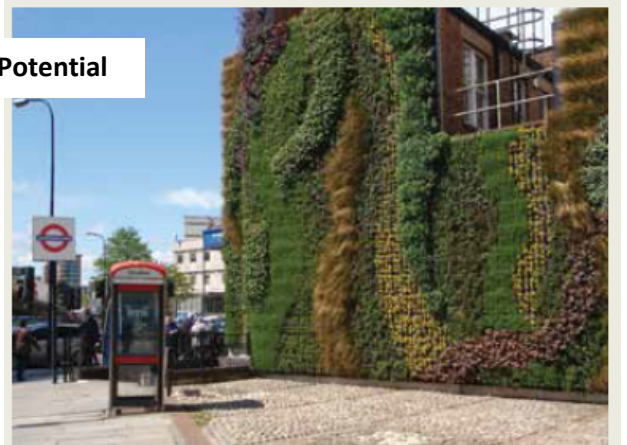
Edgware Road green wall Transport for London
